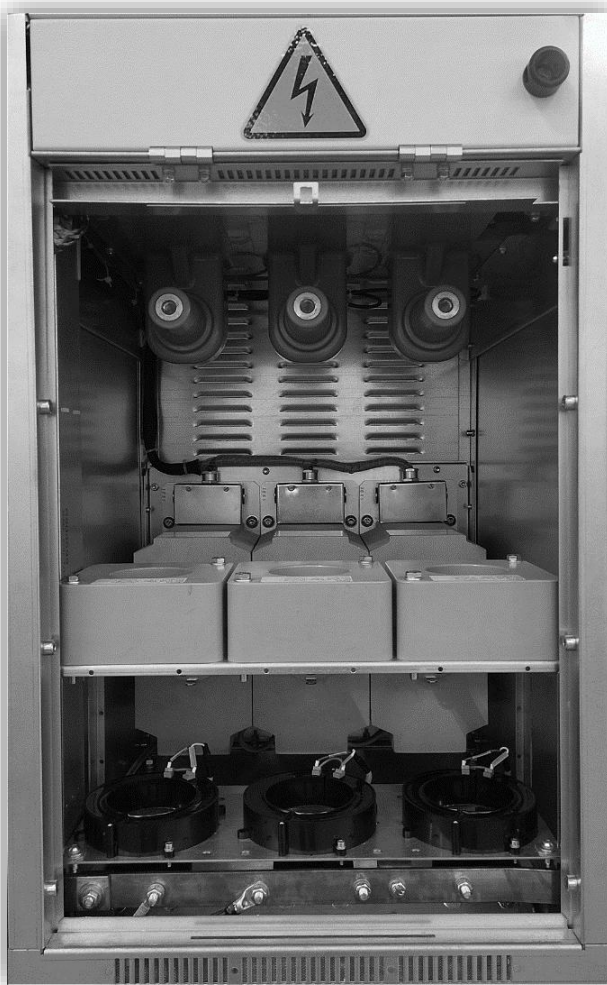
Fig.6.7. Cable compartment
